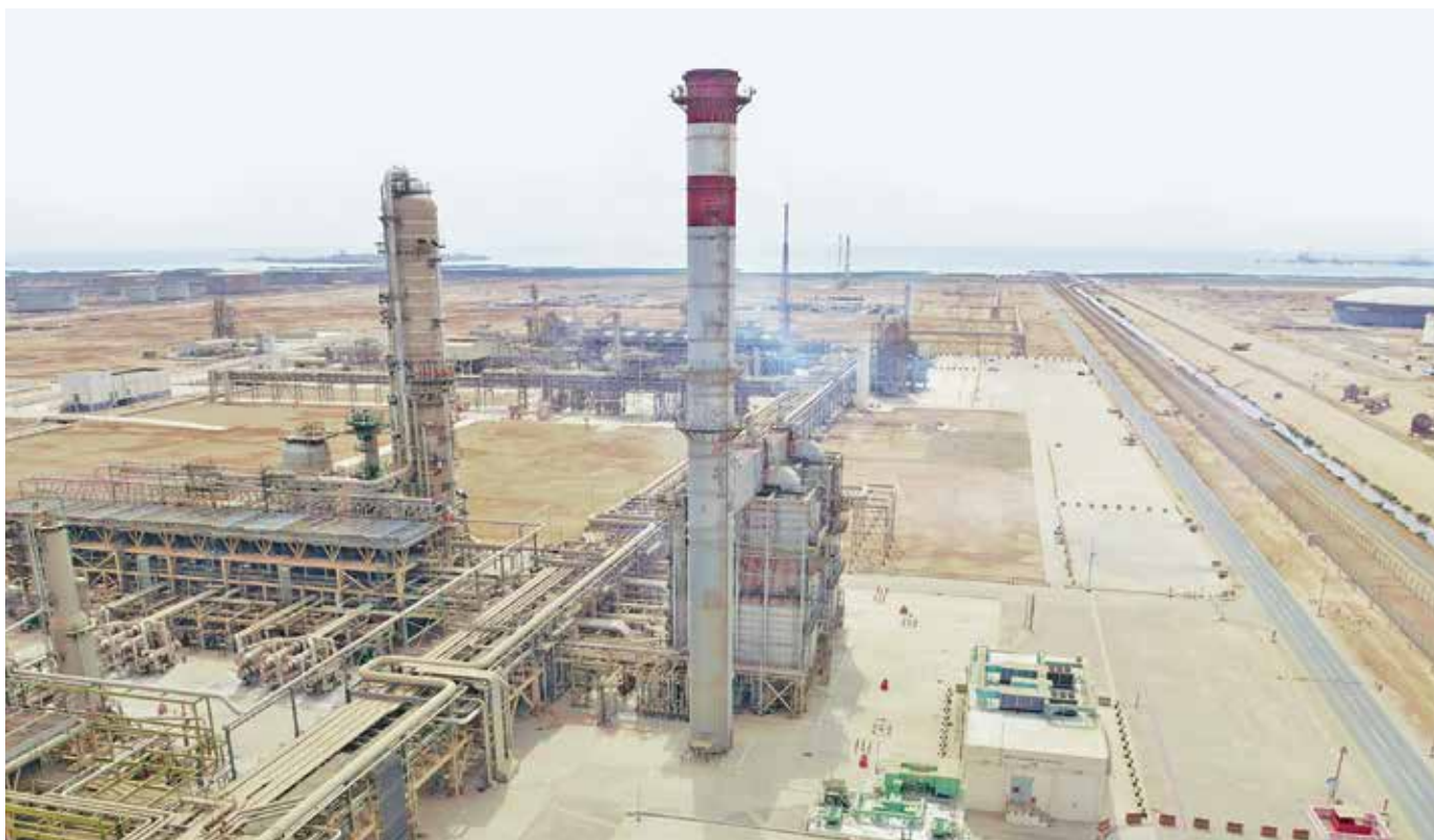
Yanbu' Refinery Department and R&DC are working to pilot a project utilizing oxy-fuel combustion, which can curb emissions. (Photo Source: Yanbu' Refinery)
