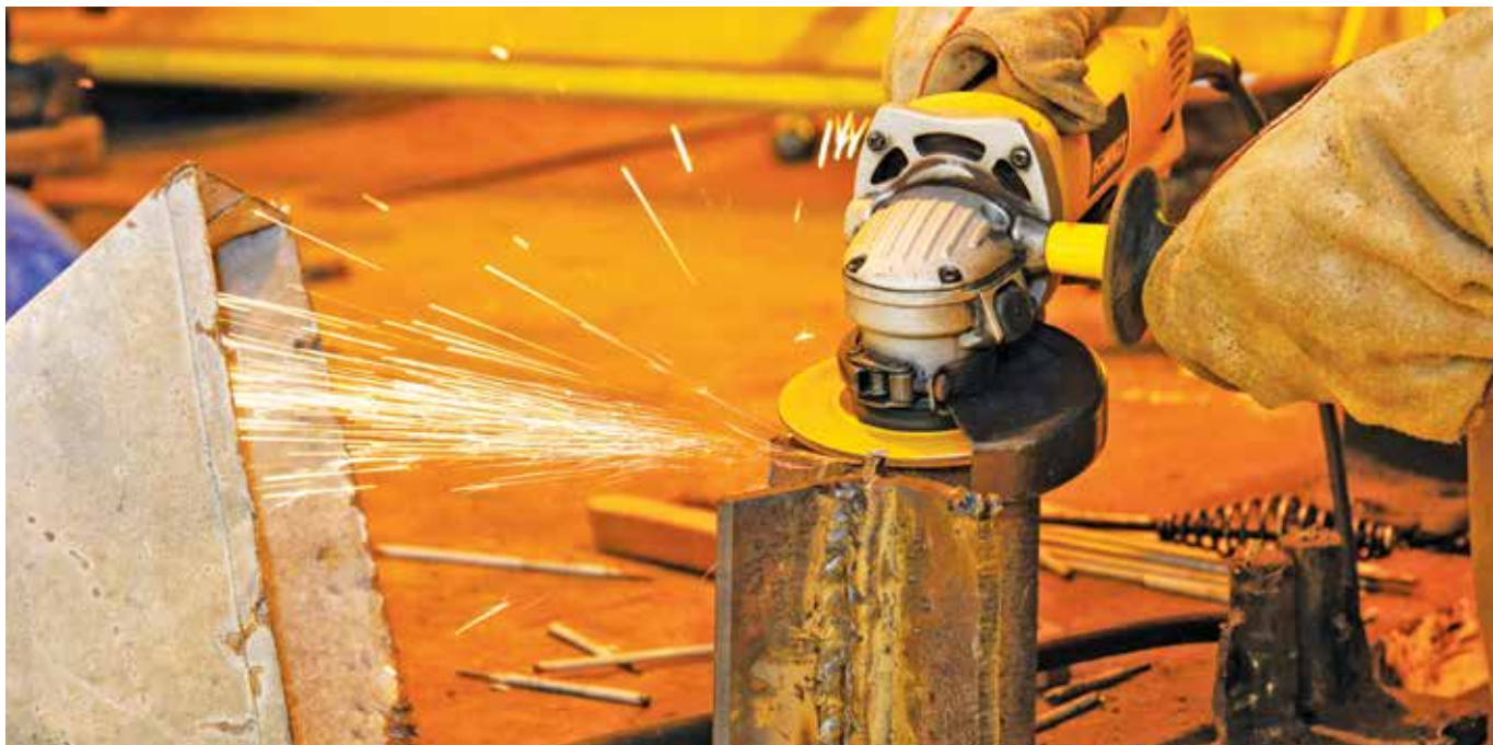
Grinding of a metal weld point takes place in a safe and properly supervised manner. (Photo Source: Saudi Aramco)
