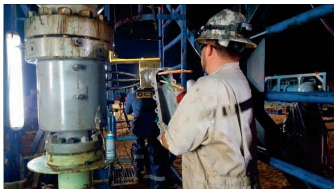
Fig. 13. Makeup of electrical connections to the cable hanger.
